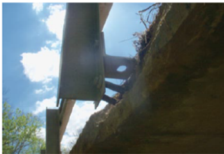
Vertical post #3 along the left side of the structure was found to be broken away from the slab.
